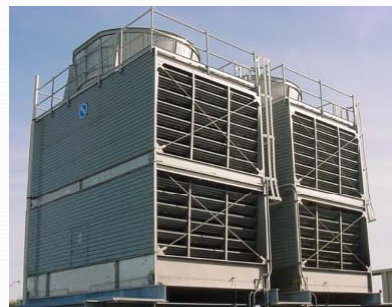
Crossflow design with double sided air inlet
