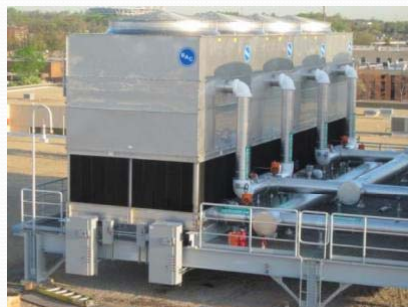
Counterflow design with four sided air inlet
